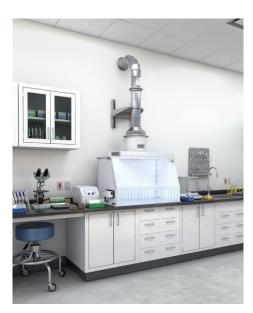
Inline Exhaust Fan attached to Ducted Fume Hood in a lab setting
