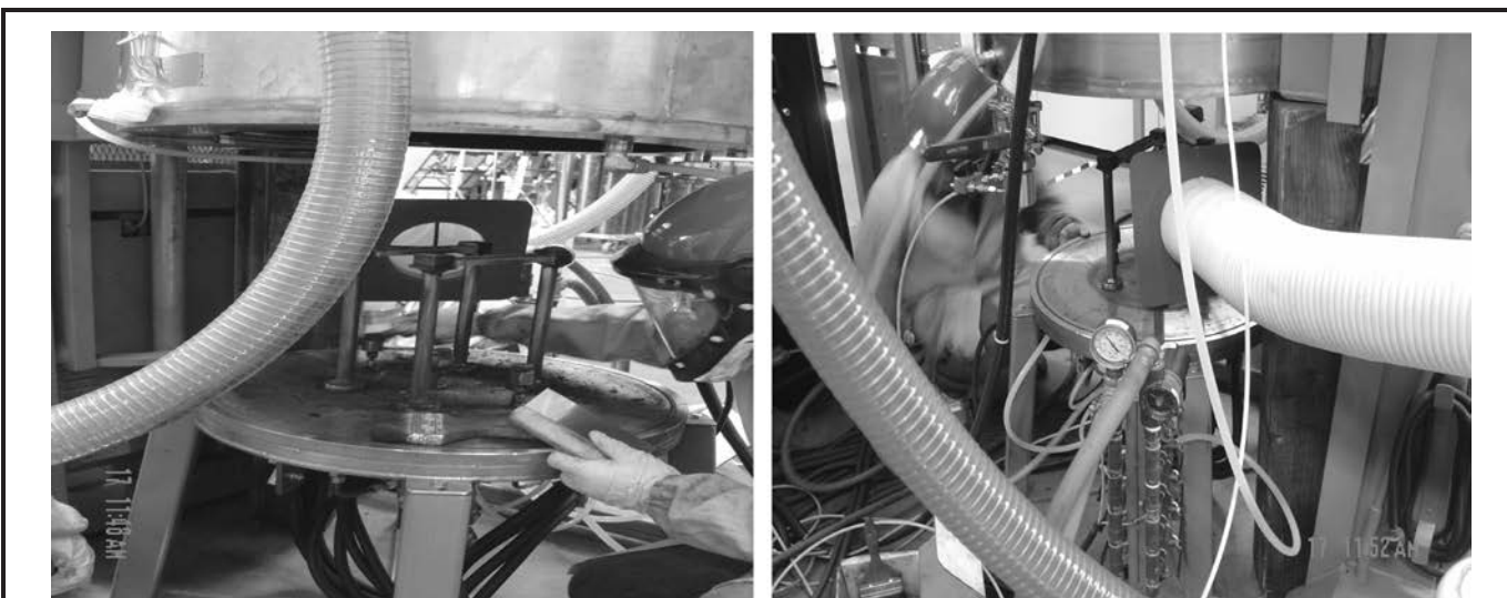
FIGURE 3. Typical location of fume extractor and production operator during reactor cleanout activities (filter-based air sampling devices located in upper left corner of photo on left)
